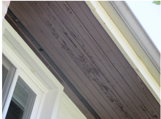
Soffit deterioration
