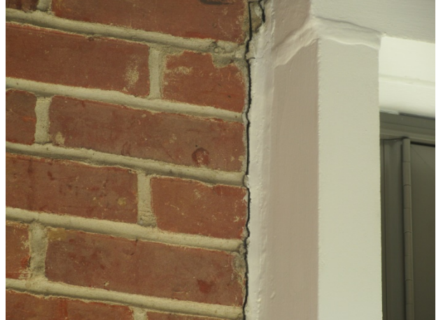
Sealant cracks
