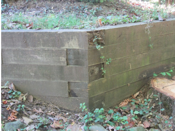
Timber retaining wall
