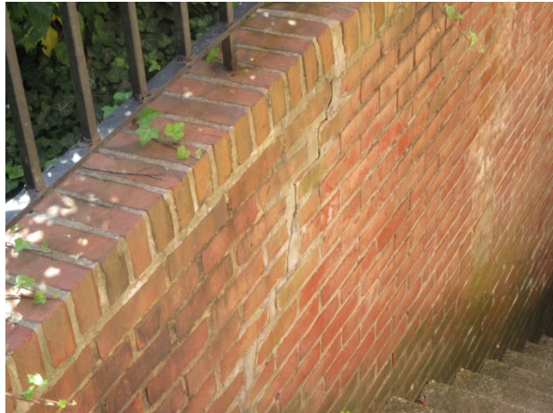
Retaining wall previous repairs
