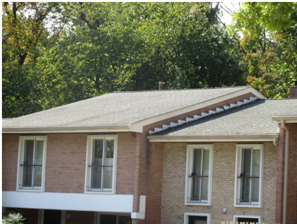
Asphalt shingle roofs
