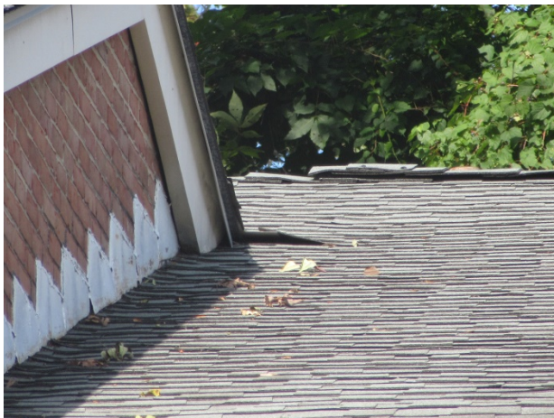
Asphalt shingle lift
