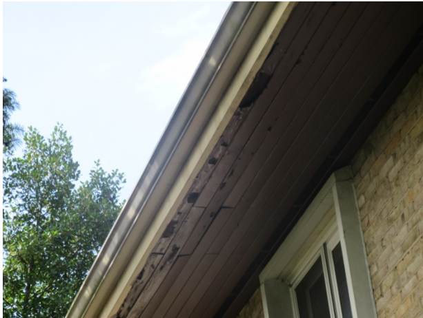
Soffit deterioration
