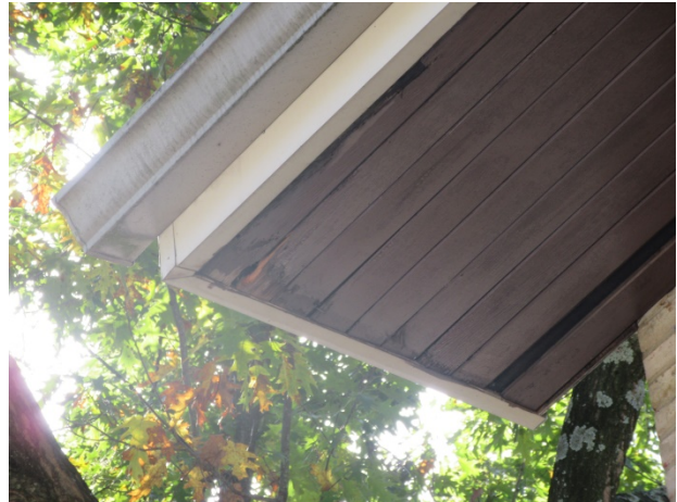
Soffit deterioration
